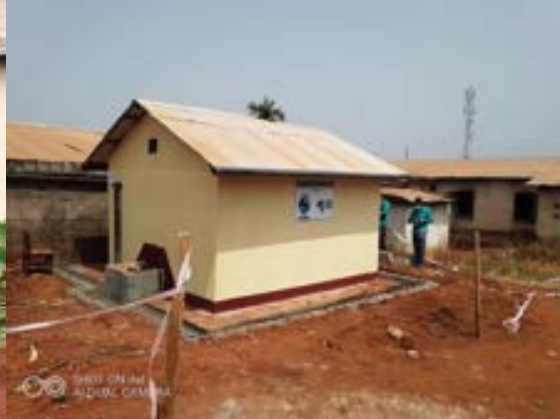
6 room VIP toilets constructed
