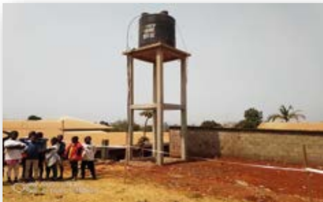
5000l water tank and stand provided
