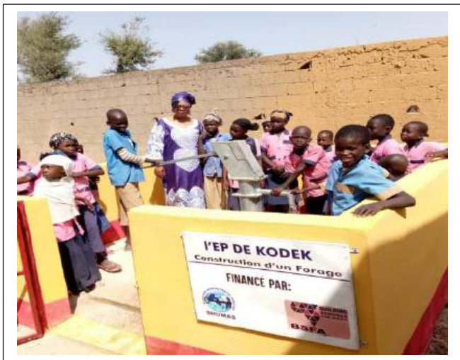
Borehole after construction
