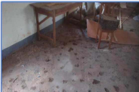
State of the floor before
