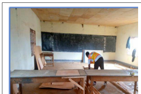
State of the ceiling after
