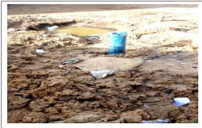
Space mapped for construction of borehole
