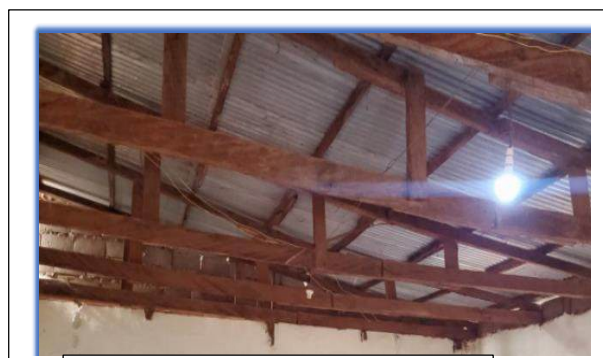
State of the ceiling before
