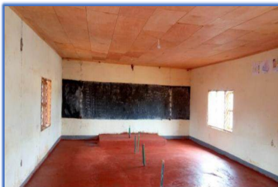
State of the floor after
