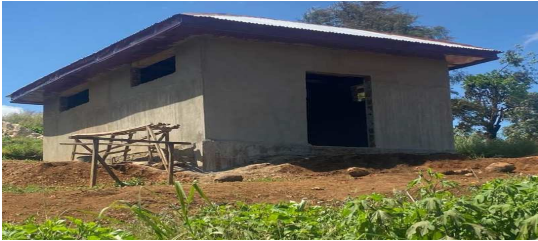
Warehouses at plastering level
