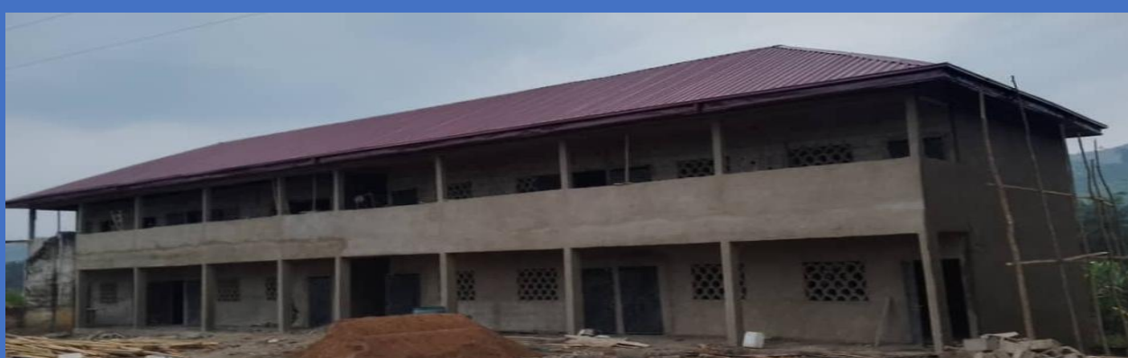
8 Classrooms, ground and 1 st floor plastered.
