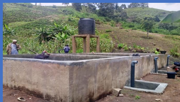
Constructed concreted fishponds with well, tank and tower
