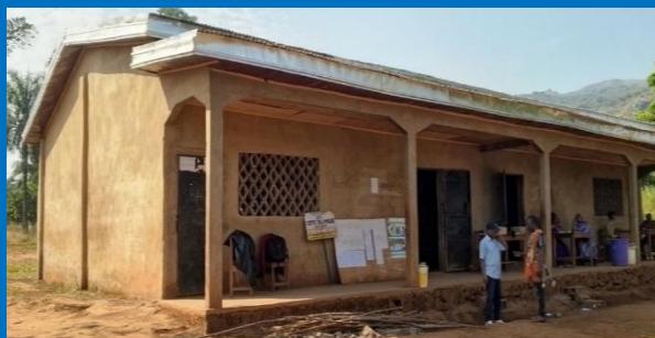
Lone structure of 2 classrooms hosting more than 300 students
