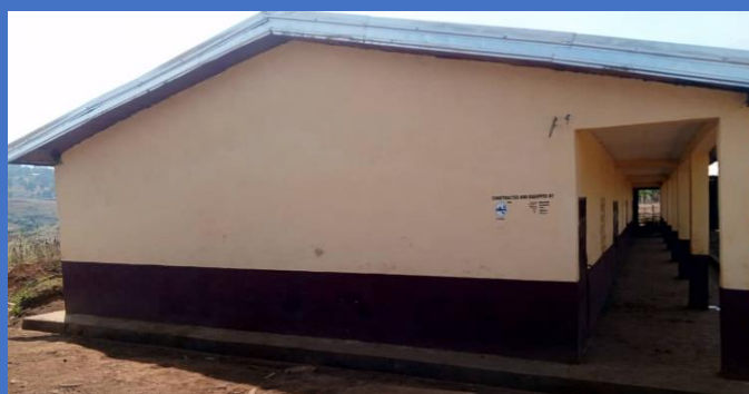
Three newly constructed classrooms.
