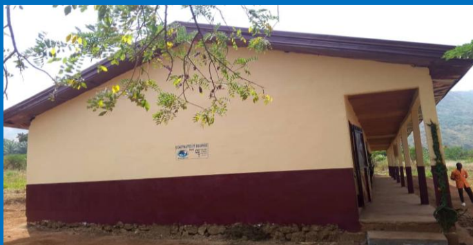
Three classrooms constructed with HT office
