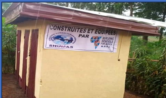
3 compartment Toilet block
