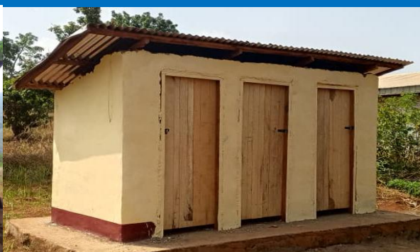
3 compartment VIP gender segregated toilet block.
