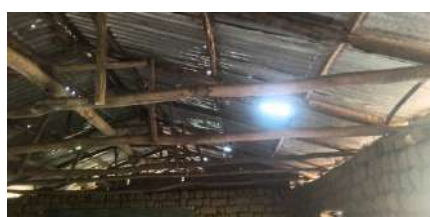
Classroom roof before
